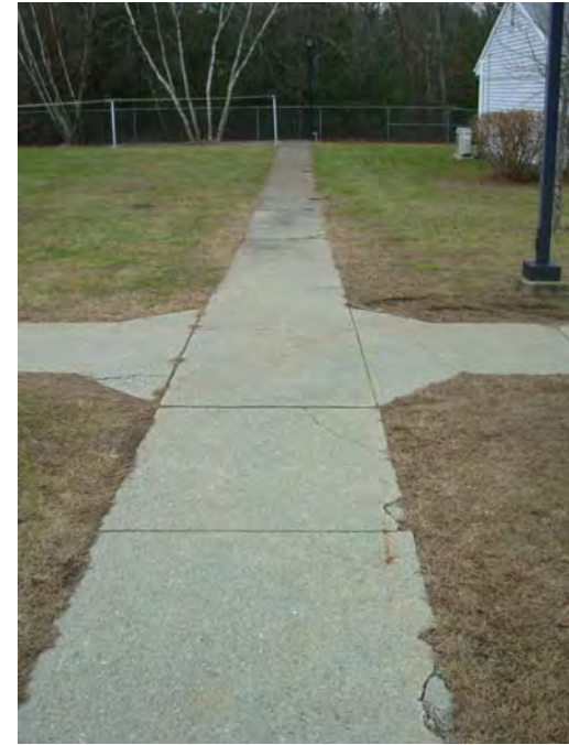
2. Spot cracking of concrete walks
