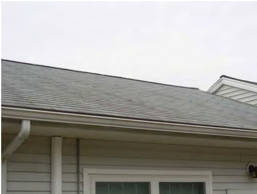
9. Staining, curling, spot lifting of roofing shingles
