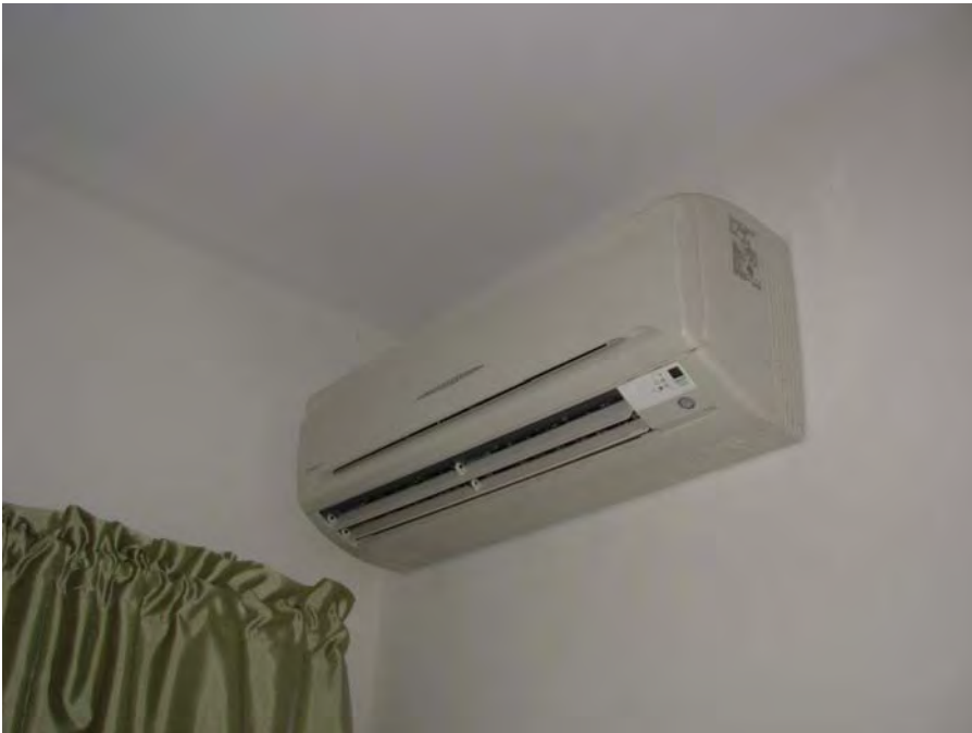
15. Heat pump HVAC systems serving units Birchwood Terrace • Capital Needs Assessment • © On-Site Insight
