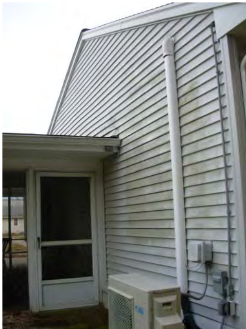
7. Spot damage and organic mtl. growth on vinyl Birchwood Terrace • Capital Needs Assessment • © On-Site Insight
