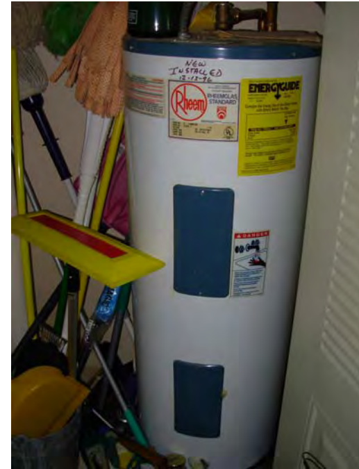
14. Typical unit DHW tanks
